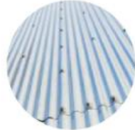
Profiled metal roof
