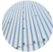
Profiled metal roof
